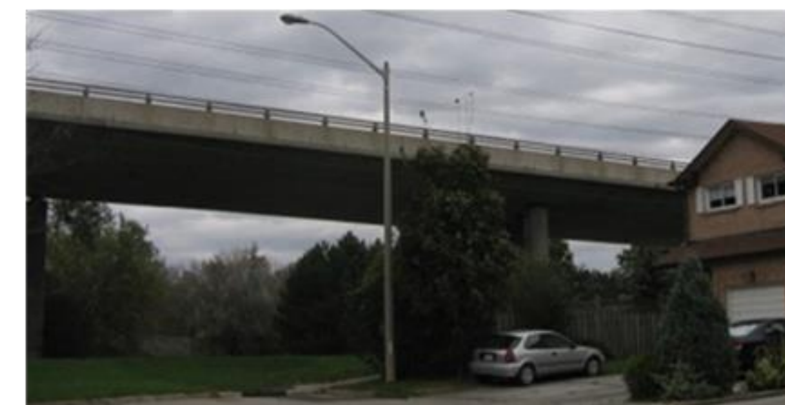
Overpass example on Bayview Avenue south of Highway 401
