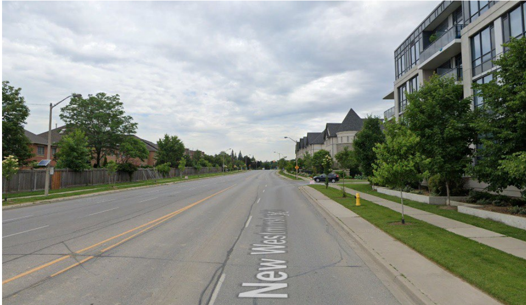
Figure 6-6 New Westminster Drive North of Centre Street
