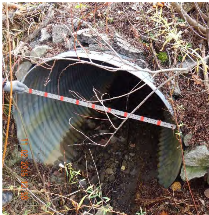
1200 mm CSP culvert between Reaches EPC-2 and 3.
