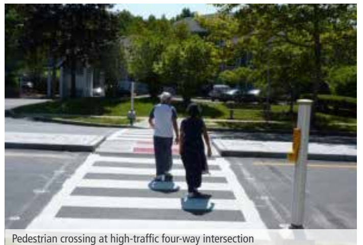
Distinctive paving to clearly define pedestrian crossings
