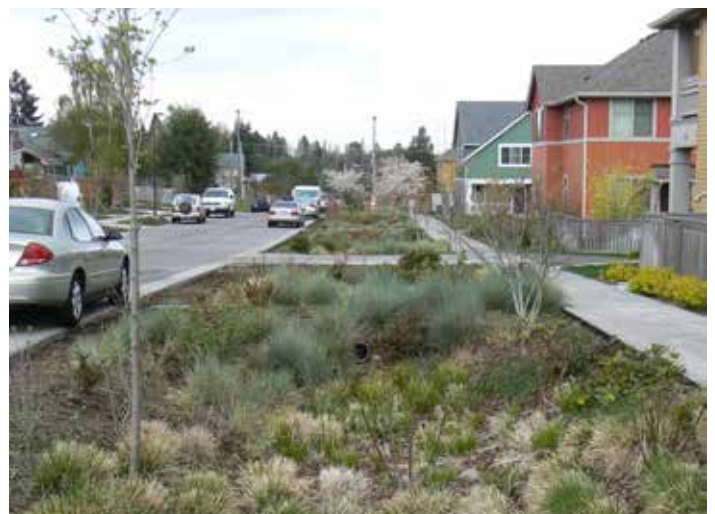
Bioswales can be integrated along roads, planted with native plants that absorb large quantities of water.
