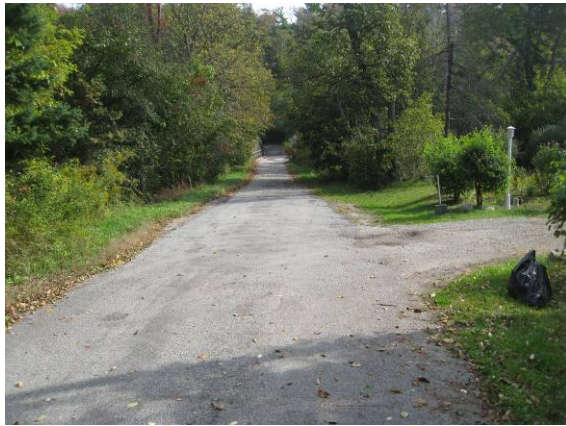
Plate 1: View northeast along Humber Bridge Trail. Note Bowstring Arch bridge in distance.
