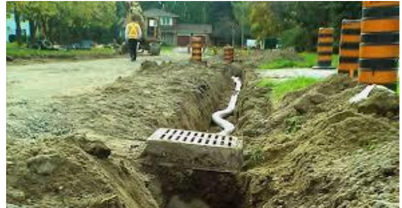
New catchbasin installation
