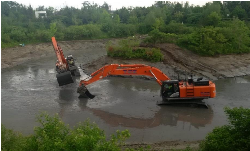
Stormwater management pond dredging to remove captured sediment
