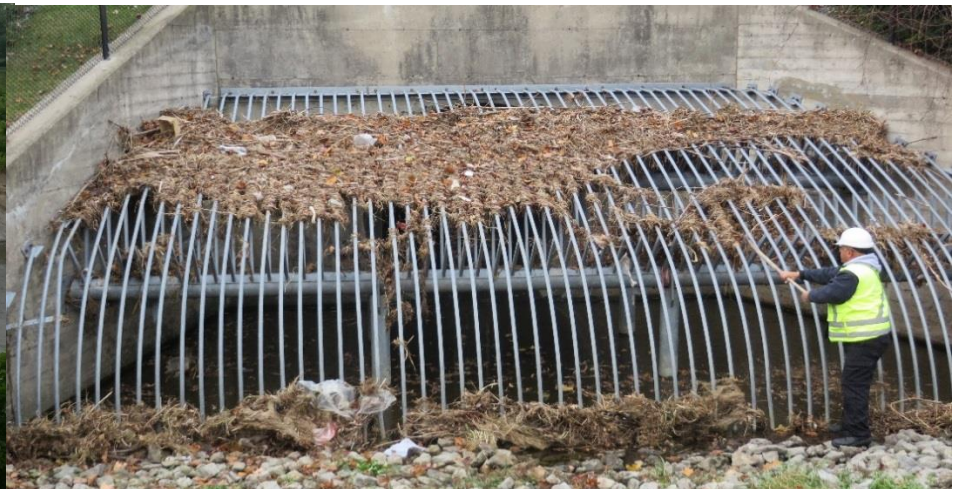
Stormwater inlet safety grate cleaning after runoff event
